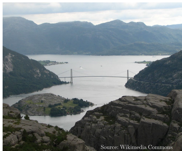
Fig. 1 East view of the Lysefjord Bridge site
