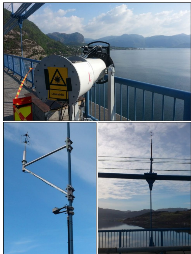
Fig. 3 WindScanner R2D1 (top) aiming at the South-West side of the Lysefjord Bridge, and sonic anemometers (bottom panels) installed above the bridge deck
